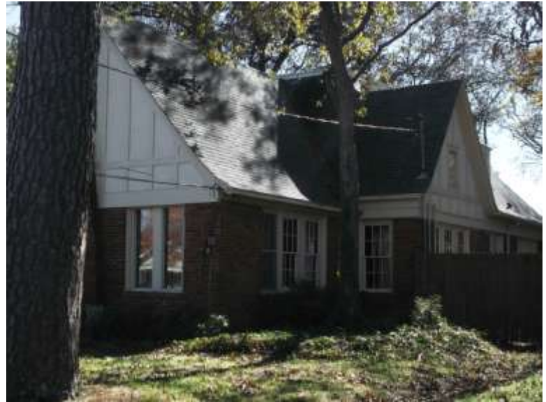
West side of house
