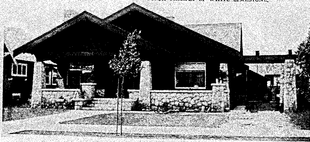
$3,000 HOUSE OF WOOD AND STONE, SHOWING COLOR SCHEME OF BLUE-BLACK WOODWORK, WITH WHITE IN STONWORK AND TRIMMING.
