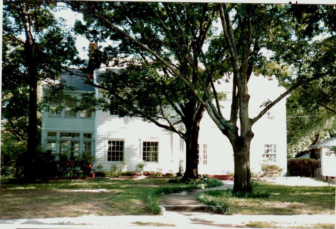
Front of house (faces North)
