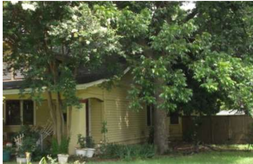
East side of house
