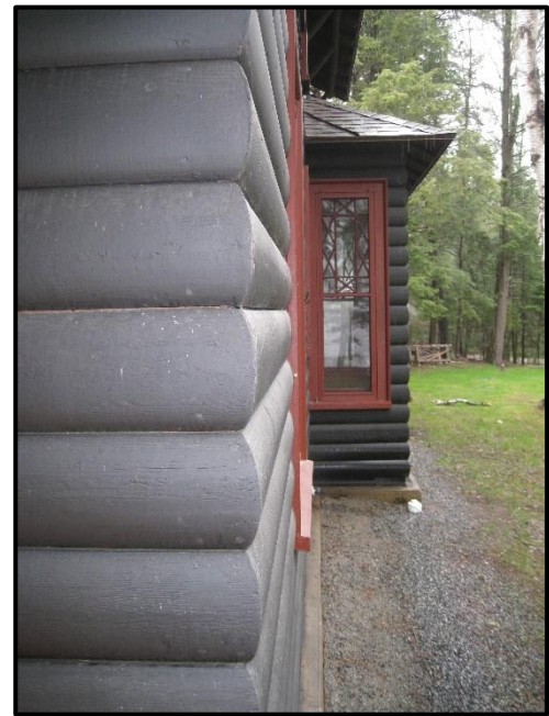
Figure 3. Mitered corners of log trim, southeast corner, 2017.
